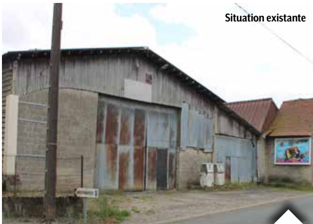
Ancienne station service, rue Roger Castel
